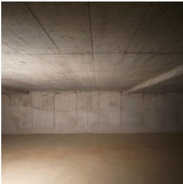
White tub concrete structures (in garages)
