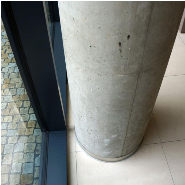
Glazed walls and visible RC elements in parter
